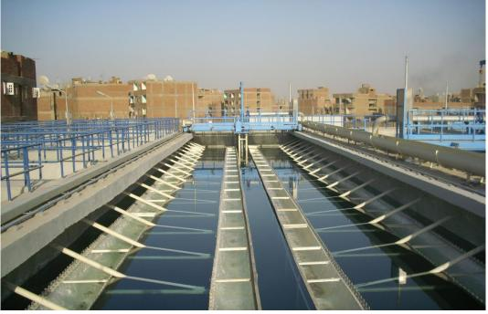
BAMAG was charged with planning, supply and installation as well as commissioning for the EI Marg potable water treatment plant which has a capacity of 600,000 m<sup>3</sup>/d.
